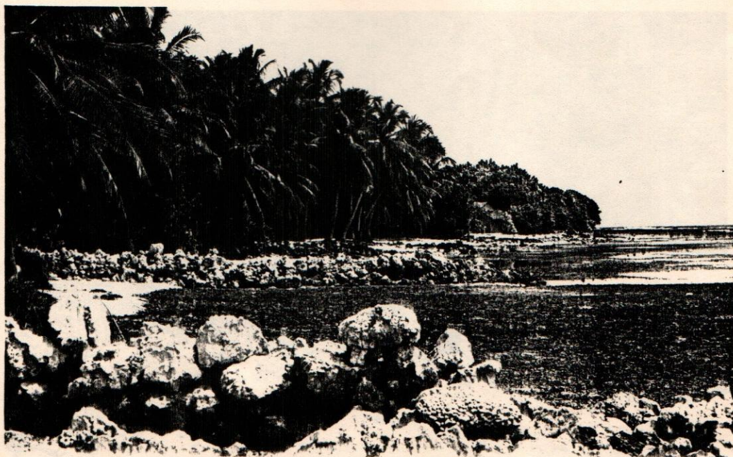
Plate 6 - Efforts to limit beach erosion using groynes in the widening channel between Hulhudhoo and Herethere have proved largely ineffectual (fig. 6-B). Complete blockage of the channel is being considered.
