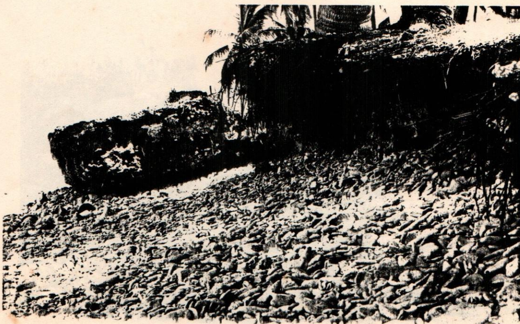
Plate 2 - Beach erosion at the RAF gun emplacement on Meedhoo (fig. 6) is due to several factors including aggregate mining, coral rubble removal from the reef rampart, and storms.
