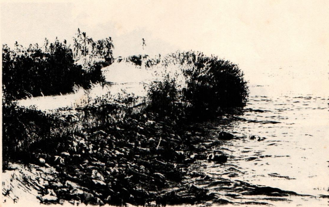
Plate 4 - The Maradu end of the Maradu-Hankada causeway is in serious danger of undercutting and collapse and the bank should be shored up.
