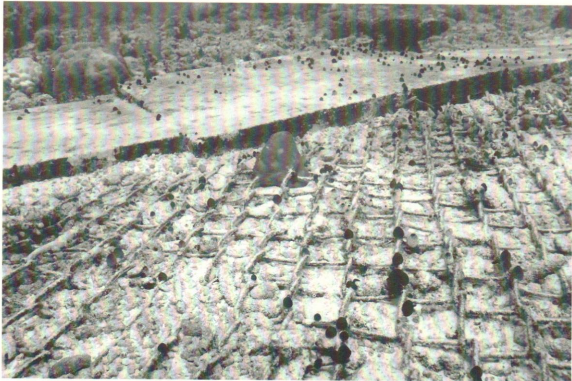
Figure 9. Chain-link fencing anchored with concrete paving slabs showing the first signs of coral growth.
