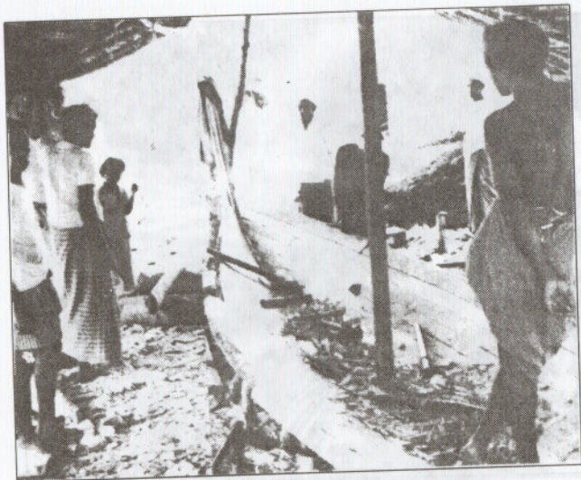
17. A small boat in the planking up stage (Photograph by Mr. H. A. Artington Davy).
